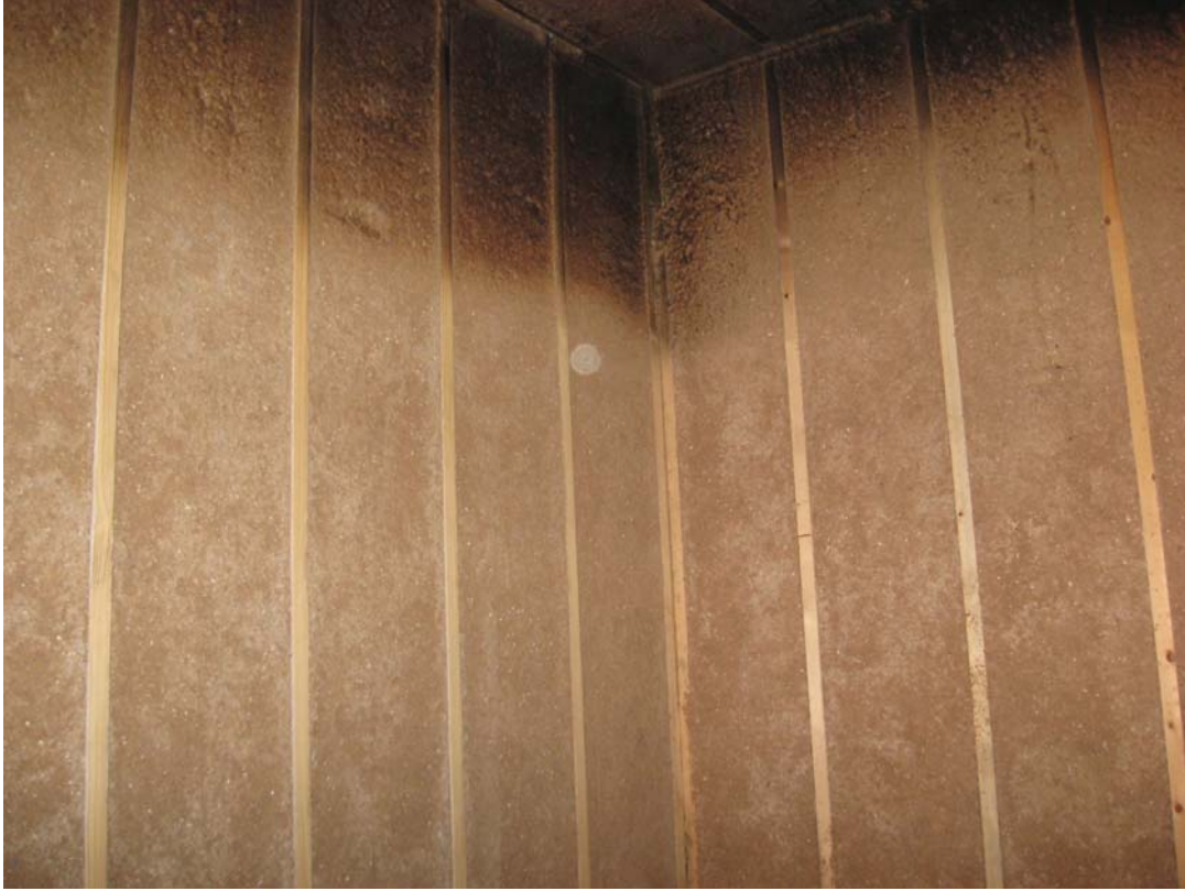
Post-test left corner.
